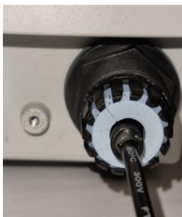
Figure 8: View of the rubber placement
