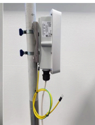
Installation the Wirnet™ iStation on the support
