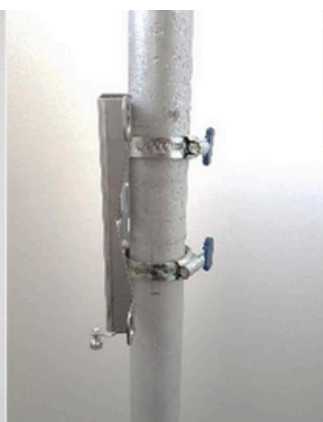
Installation support on a pole with strapping
